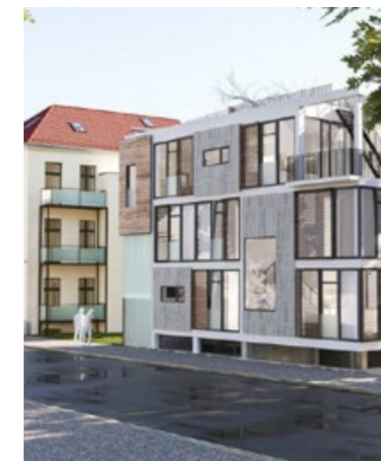
Am Langen Felde, Leipzig New construction and core renovation of a listed building from 1880.
